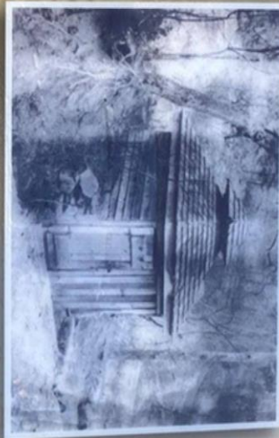
The present stonework may date back to the 18th century. Around 1915, forestripes removed the front wall of the stonework enclosure and built a wood frame springhouse to keep the water clean and cool. An iron grate was added during the 1930s. The current springhouse is a reproduction of the original structure, which stood atop the stonework and pool.
